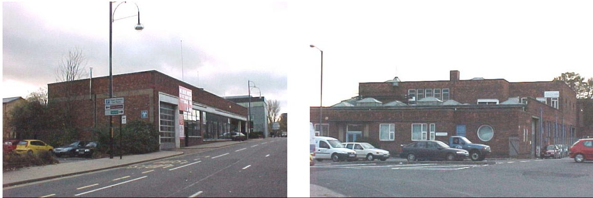
Former Kwik-Fit building and ACC Dairy
