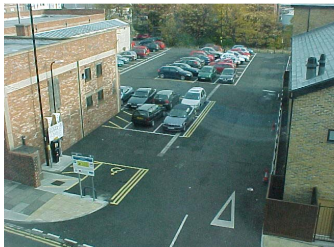
Car Park between the Baptist Tabernacle and former Kwik-Fit, looking east.
