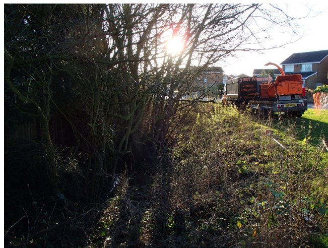
Surbiton Road – December 2014 (before work)
