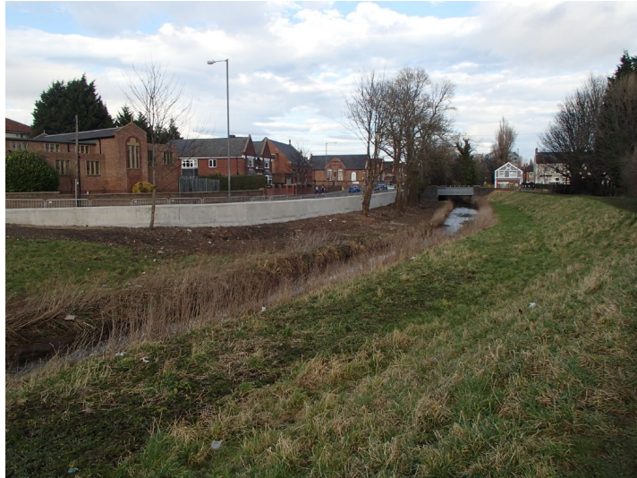
Bishopton Road – February 2015 (New flood wall)
