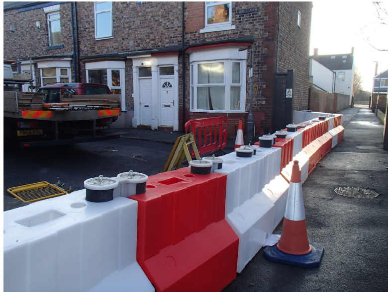
Stockton Council Flood Barriers at Bedford Street, Stockton
