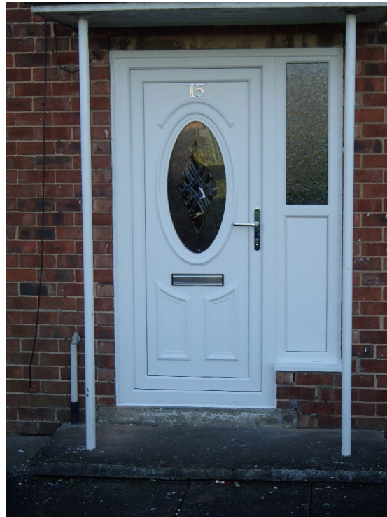
Ilkeston Walk, new flood door – April 2015
