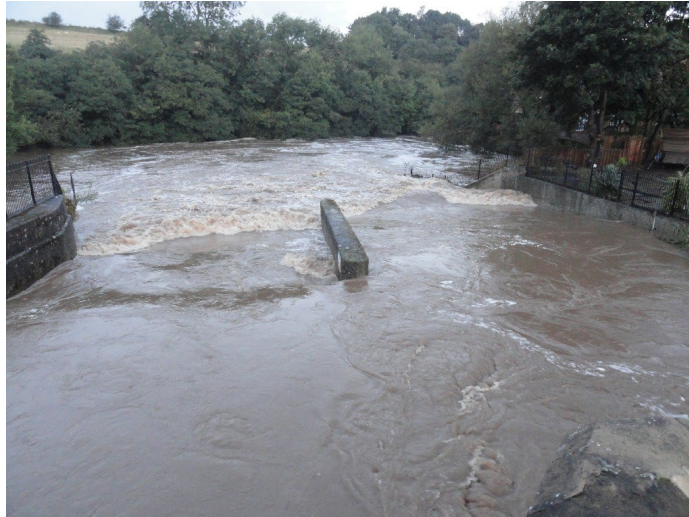
Leven Bridge – September 2012
