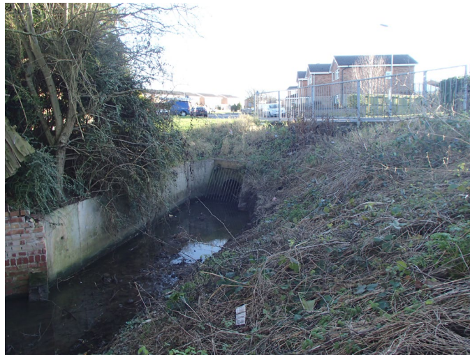
Surbiton Road – January 2015 (after work)
